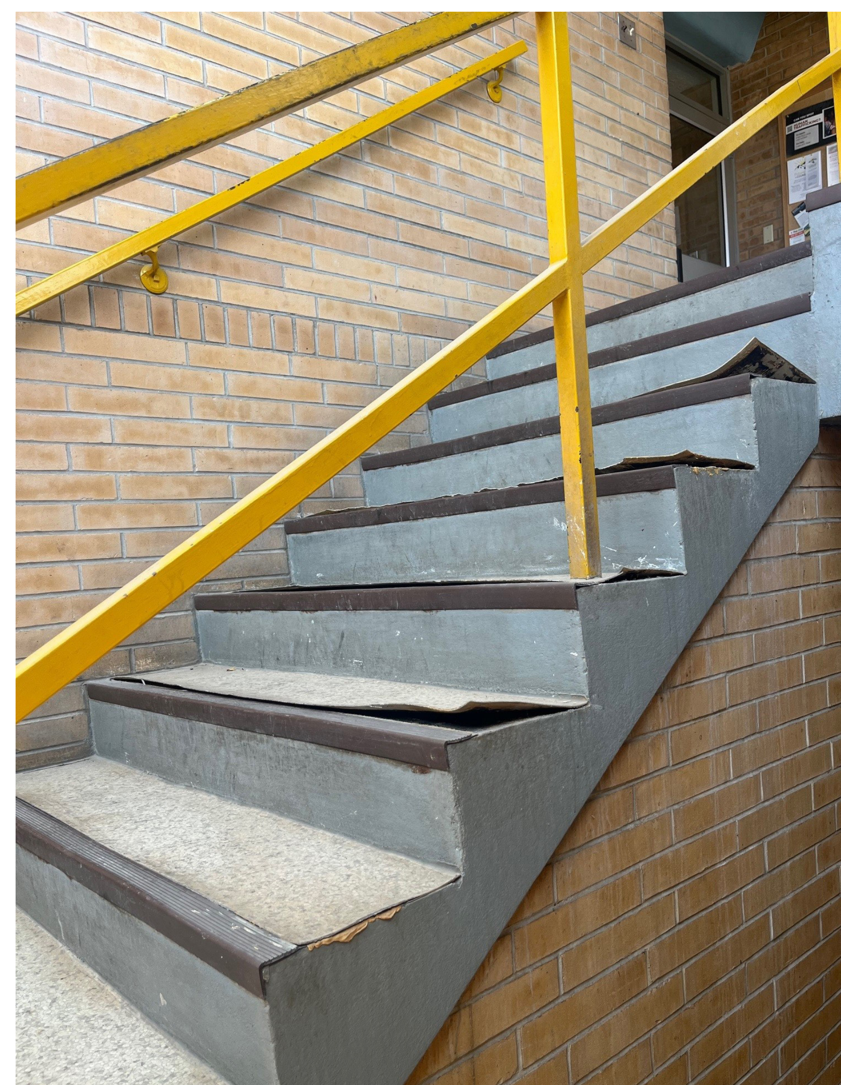
Damaged stair tiles
